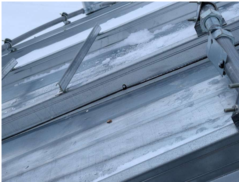
Figure 3. Wiring Picture with Self Tapping Screws and P-Clips
