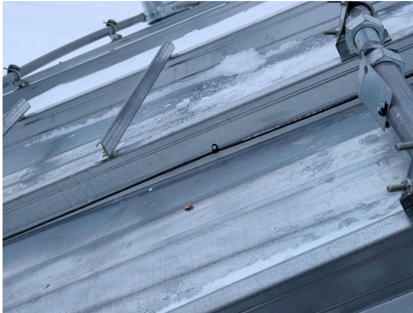
Figure 5. INT2 Secured on Bin Roof With P-Clips
